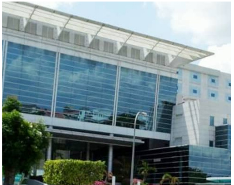
PUBLIC BANK IT & TRAINING CENTER
